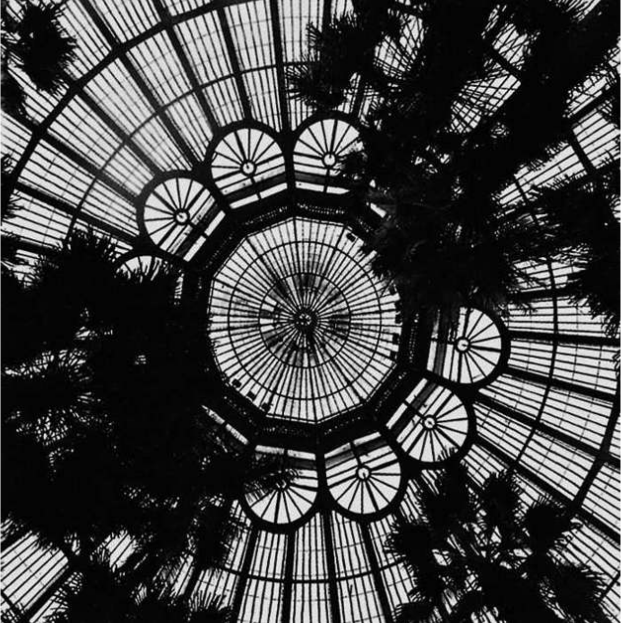
View of the roof structure.
