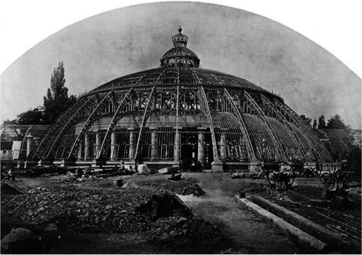
Greenhouse in the park of Laeken Palace, near Brussels, during construction, 1875.
