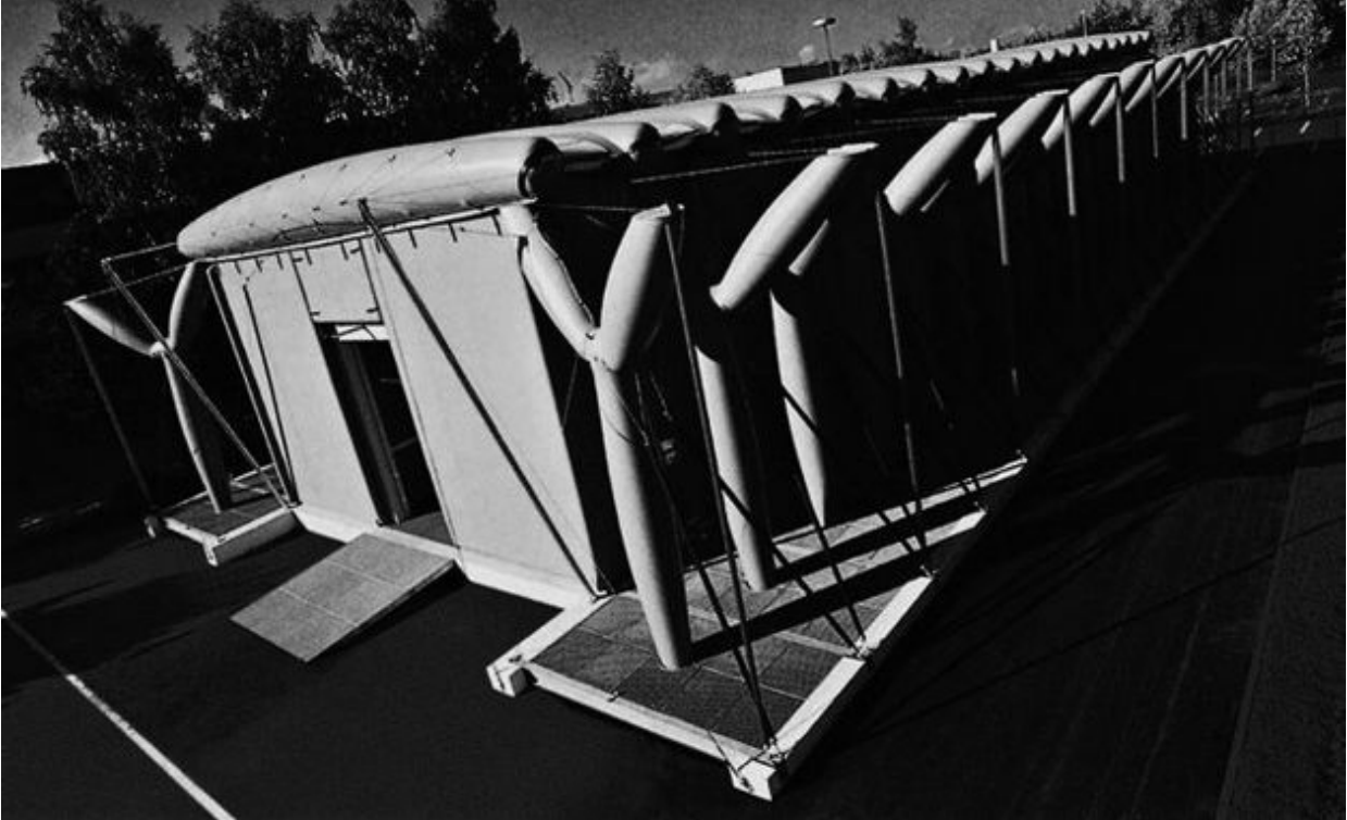
Axel Thallemer for Festo Corporate Design, Airtecture Hall , 1996. Air-filled roof beams and Y-shaped side supports, material: vitroflex covering.
